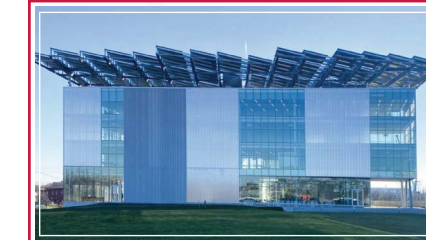
ENERGY ADVANCEMENT & INNOVATIONS CENTER
