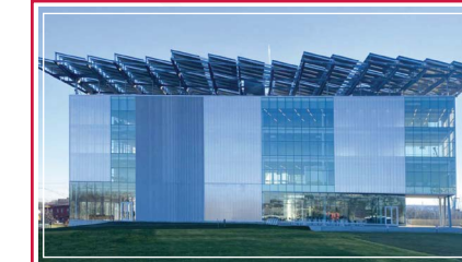
ENERGY ADVANCEMENT & INNOVATIONS CENTER
